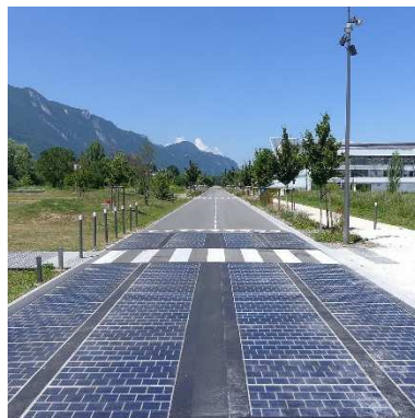
Portion of a solar powered road in Savoie Technolac science and technology park - Savoie (France) Source: Wikimedia (Florian Pépellin - licensed under CC-BY-SA 4.0)
