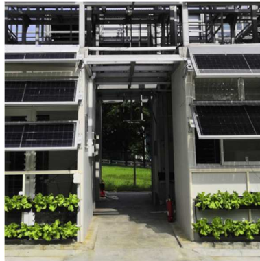
Mockup of productive façade Source: Tablada et al. 2018
