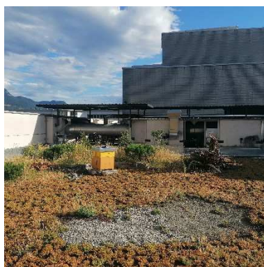
Extensive green roof, Bolzano (Italy) Photo: S. Croce
