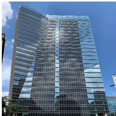
BIPV façade - Gioia 22, Milano (Italy) Photo: M. Formolli
