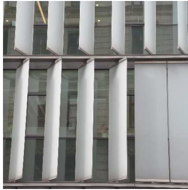
Vertical louvres applied on an office building - Vienna (Austria) Photo: S. Croce
